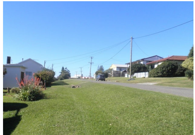
Figure 7 - Storm water swale in Lindsley St
